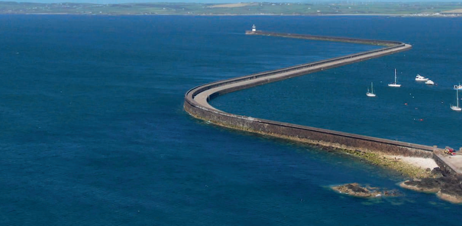
Aerial view of Holyhead Breakwater, with almost 2.39 km the longest of its kind in Europe. Construction on the embankment foundations began in 1847 and took 26 years to complete. Over 1,500 men were employed to build it.
