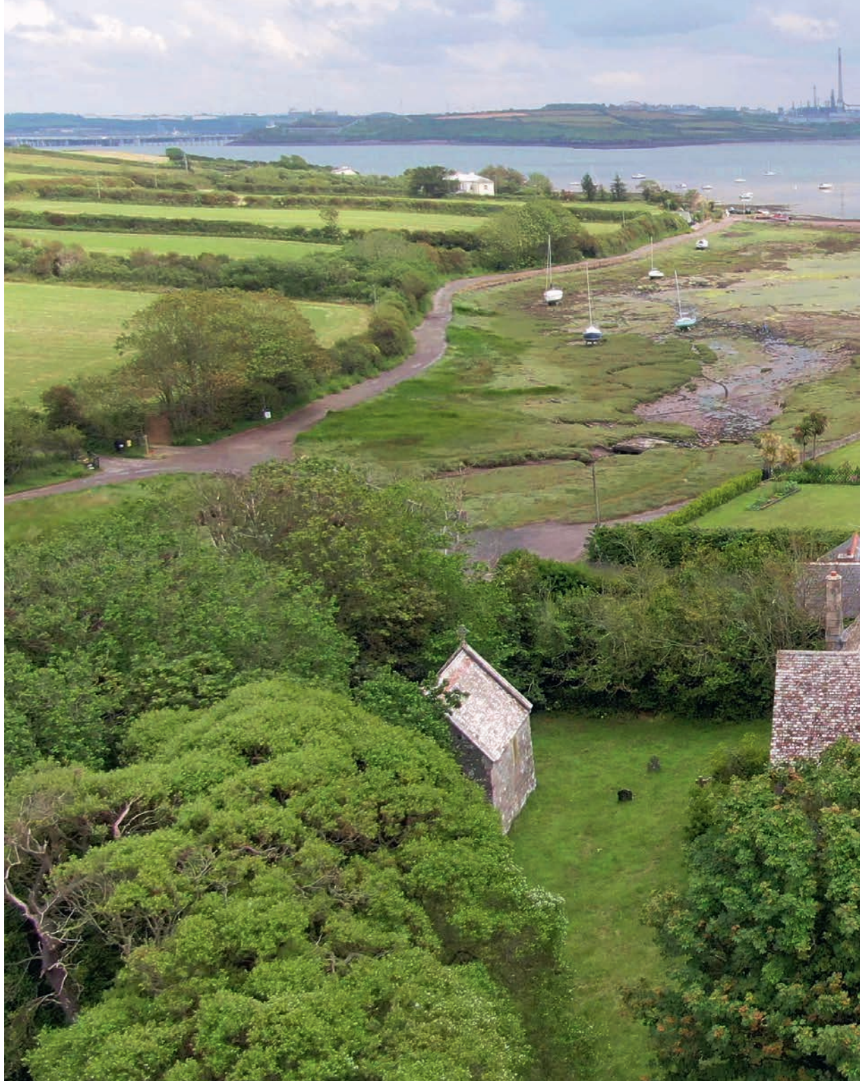
Aerial view of St Mary's, Angle, towards West Angle Bay and the Milford Haven Waterway.
